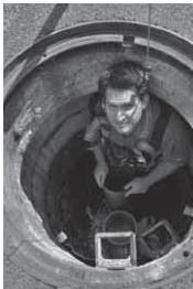
6. Go down into the shaft and position on the filter elements
