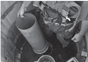
1. Pull the overflow out of the bushing and lift it out of the shaft
