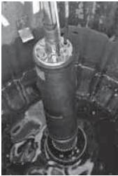
1. Lower the pump through the outlet tube into the shaft
