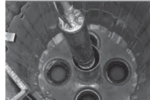
6. When the shaft is clean, the pump can be pulled out
