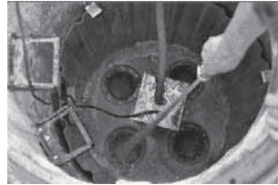
5. Flush the sealings for the filter elements thoroughly
