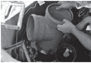
3. Take out the T-piece completely and lift it out
