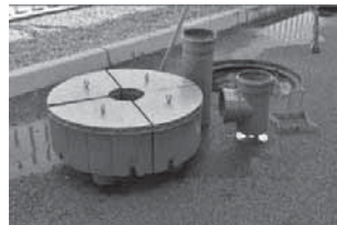
2. All is prepared for the installation of the filter
