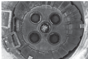
1. This is how the shaft looks now from inside
