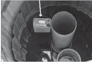
2. Check the atmosphere in the shaft with the gas detector and observe it constantly
