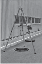
1. Position the rescue tripod above the opened shaft
