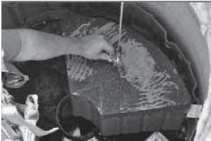
1. Hook the wire rope into the filter ear and pull out the filter completely out of the shaft
