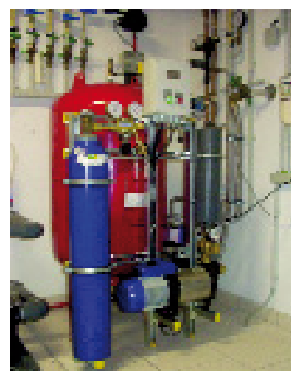
Underground water purification system UWEMAoxygen.
