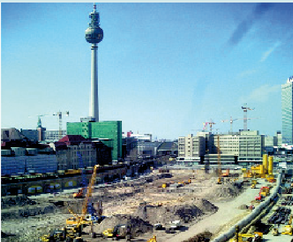
Temporary sewer bypass DN 2200 at Alexanderplatz, Berlin. Reproduced with kind permission of beton & rohrbau C.-F. Thymian GmbH & Co KG, Berlin
